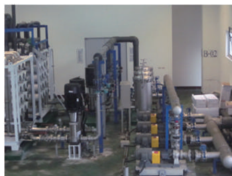
RO給水系統 RO Supply Water System
